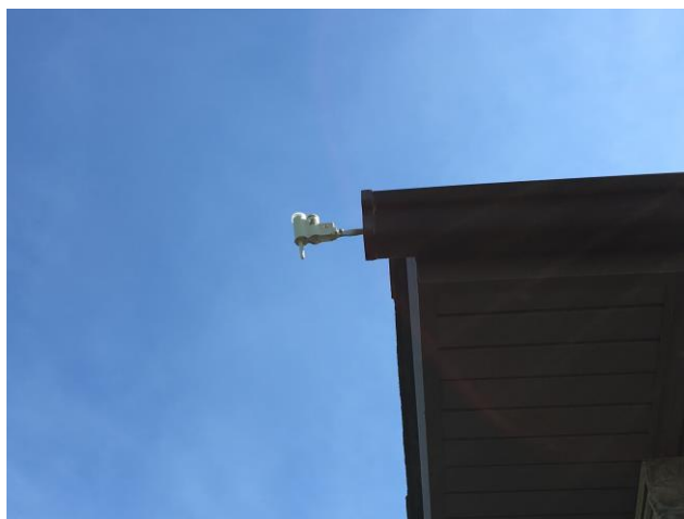
PROPER INSTALLATION OF A RAIN SENSOR
