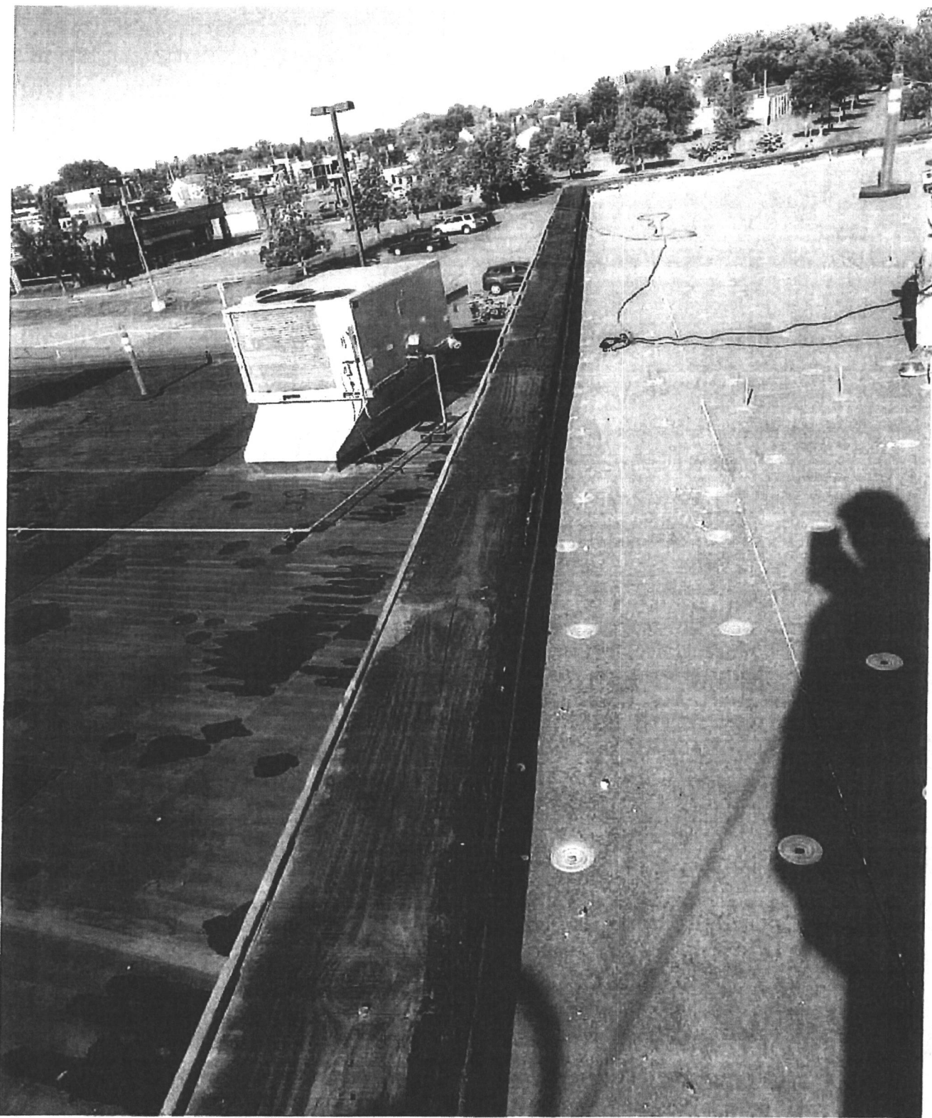
A1 - SOUTH PARAPET OVERVIEW PHOTO
