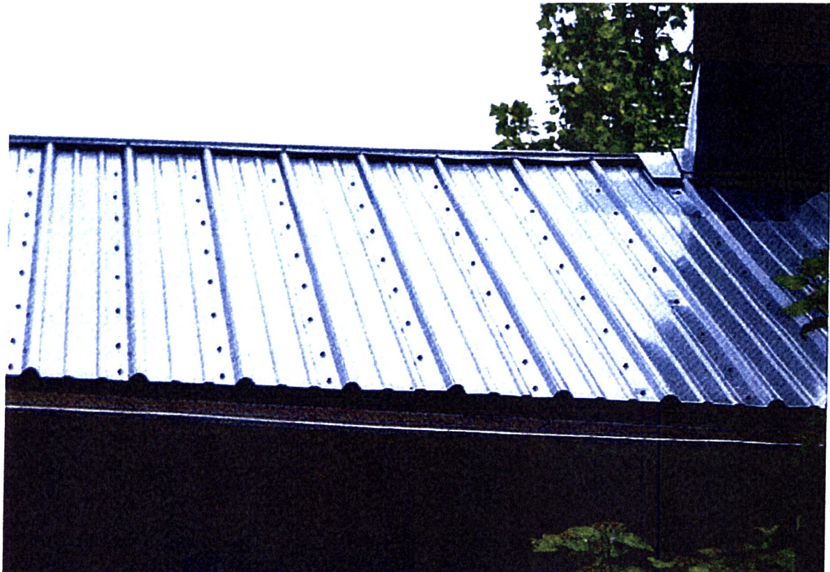
Exposed fastener metal roof examples
